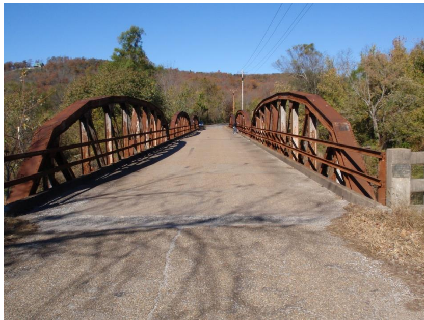
Figure 4.4: Baptist Ford Bridge – View of Bridge Deck Photo taken by Jeremy Rawn, Fall 2010 Fayetteville, Arkansas
